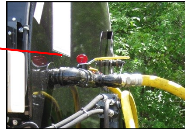
Tank Return Valve (7)
